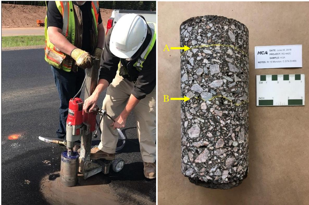
**Figure 2-6 Coring Operation Using Pedestal and Support Column (Left), Interfaces Under Study Shown on a 100-mm Diameter Core: Interface Between Newly Paved Surface Course and and Base Course Mix (Marked as “A”) and Interface Between Newly Paved Base Course and Milled Surface (Marked as “B”) (Right)**
